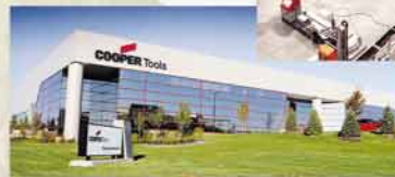
Automated Systems North American facility located in Auburn Hills, Michigan from which we provide full design and manufacturing capability.
