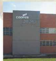
Cooper Tools Industrial Ltda. facility located in Sorocaba, Brazil.
