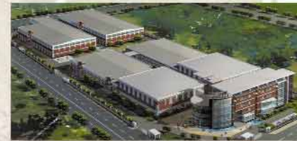
Cooper facility located in Shanghai, China.
