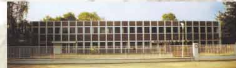
Recoules facility located in Ozoir-la-Ferrière, France.
