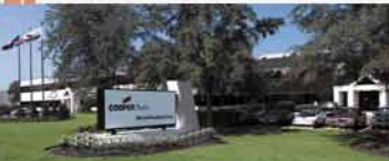
Cooper Power Tools Division headquarters and manufacturing facility, Lexington, SC.
